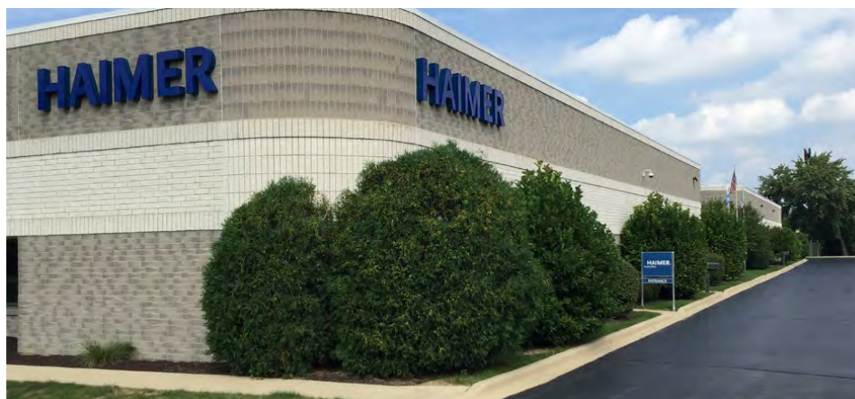
HAIMER USA and North American Headquarters in Villa Park, IL
